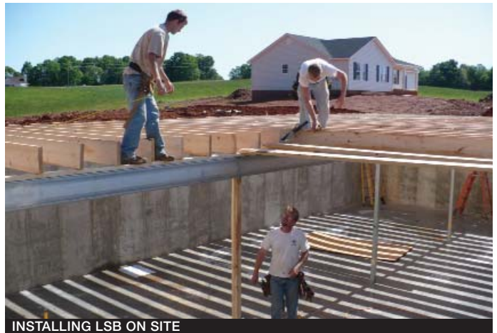
INSTALLING LSB ON SITE
