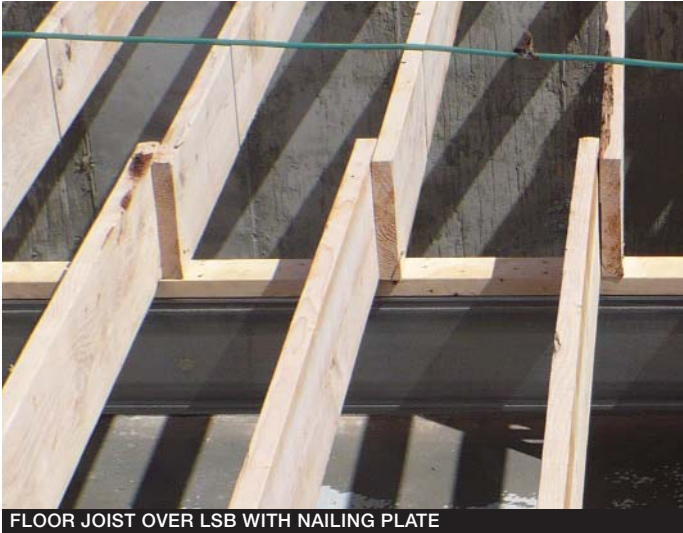
FLOOR JOIST OVER LSB WITH NAILING PLATE
